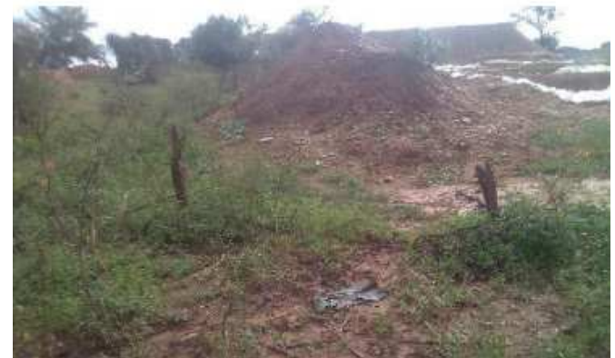
Pictorial Evidence 2: Damaged Fence at Dore Green Custom Milling
