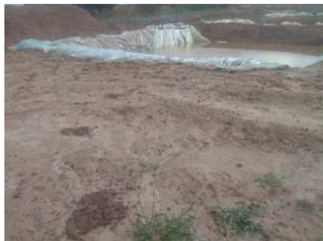
Pictorial Evidence 5: Unprotected Tanks at Dore Green Custom Milling
